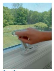
**Step 2**At the bottom of the window, pull the crank out of the pocket and turn the crank until the window is open to your liking.
