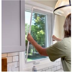
**Step 1**Grabbing both sides of the screen, push down then pull out to remove the
