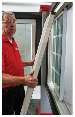
**Step 3** You can now pull the sash out of the top track and remove it from the window.
